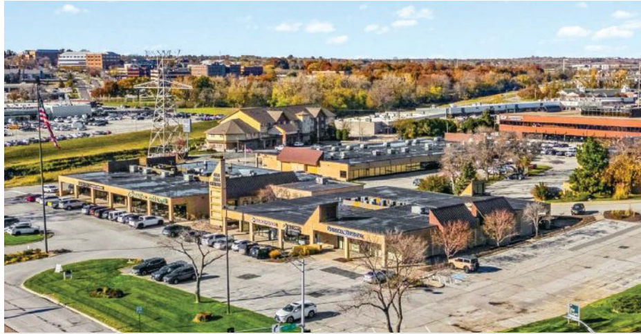
Earlier this year, Old Mill Centre in Omaha sold for $7.5 million. The 21-suite retail strip center totals 75,089 square feet across four buildings.
