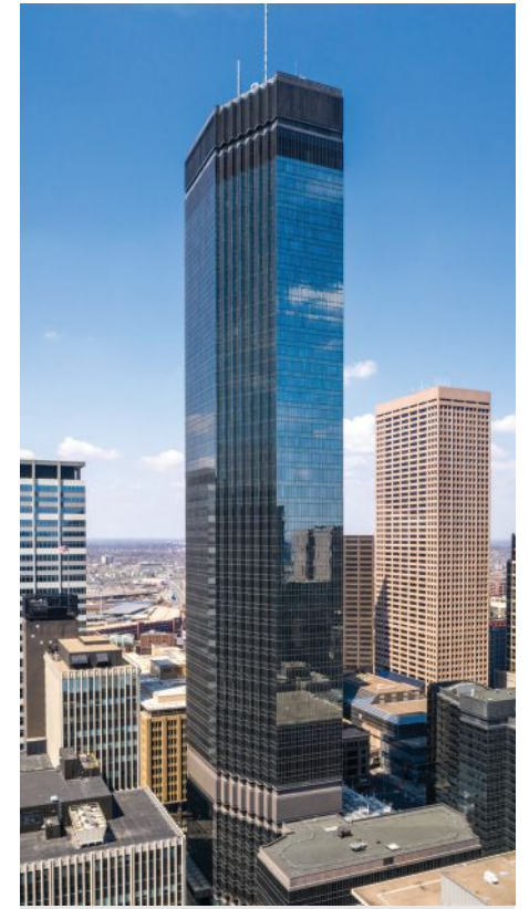
Law firm Zimmerman Reed recently signed a long-term renewal of its 15,179-square-foot lease at IDS Center in downtown Minneapolis.
