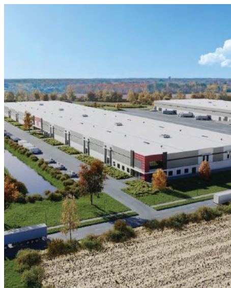
Hempel Real Estate is underway on Brockton Business Park in Corcoran, Minnesota, near I-94.
